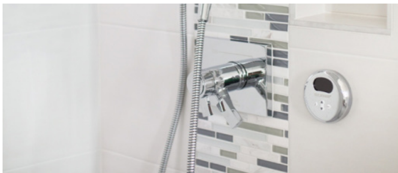
Hot water button to reduce water waste Photo Credit. Department of Energy
