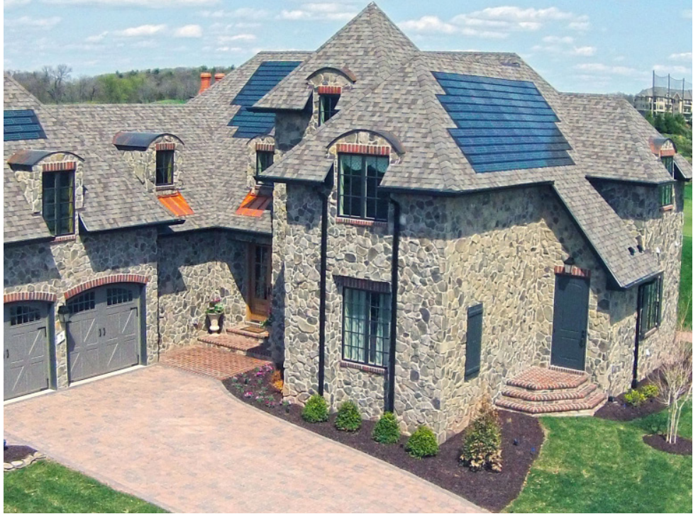
Roof-integrated photovoltaic shingles Photo Credit. U.S. Department of Energy
