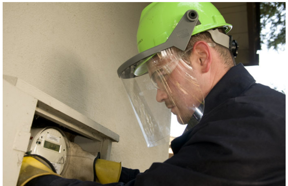
Installing a smart meter Photo Credit. pgegreenenergy / Foter / CC BY
