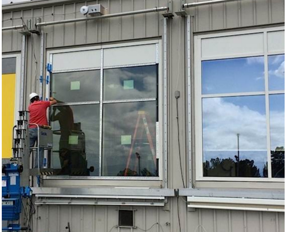
Installing energy efficient windows. Photo Credit. Department of Energy
