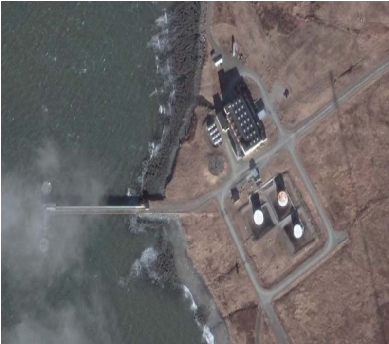
Power Plant 18 MW
