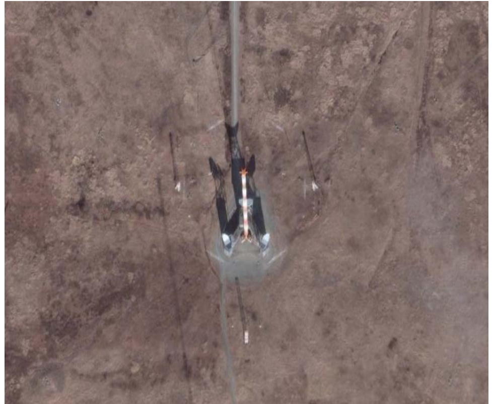
Main Tower And Helix House
