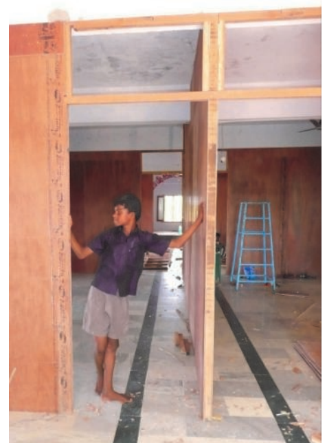
Bernard examines the workmanship.
