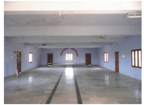
Inside the Main Building before partitions were installed.
