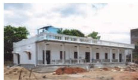
The boys' new study hall and dormitory is also near completion. It will eventually accommodate 48 boys.
