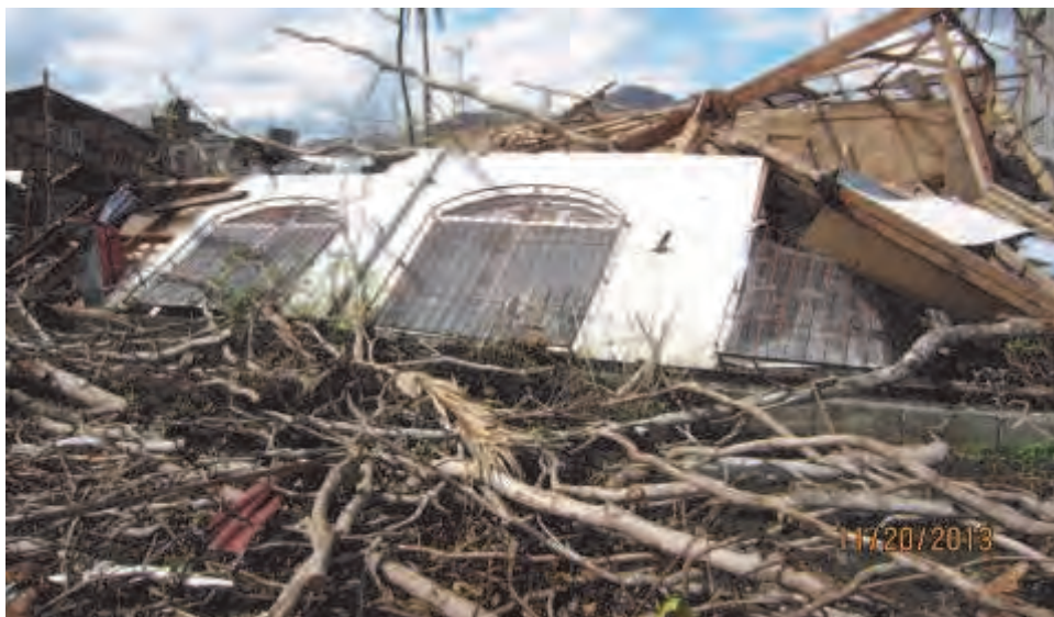
Holy Family Chapel, Tacloban, sustained significant storm damage in the typhoon....
