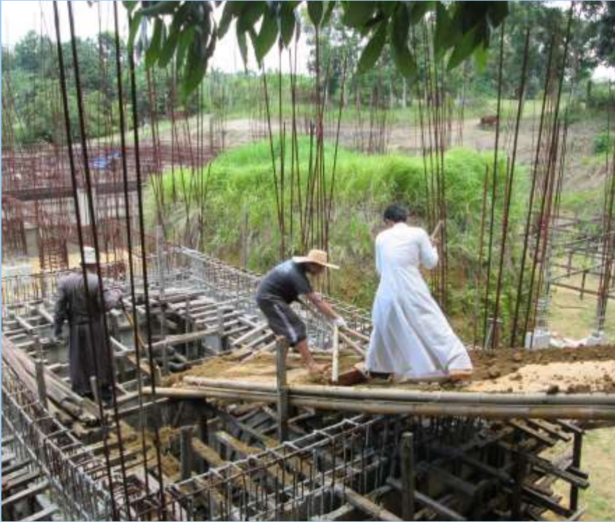
A little African-Philippine engineering! A sand-slide constructed to facilitate the refill process. The Brothers seem to find their second childhood on this slide!!
