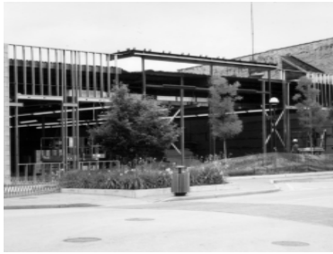
New structural steel was added to support a massive limestone frontispiece.
