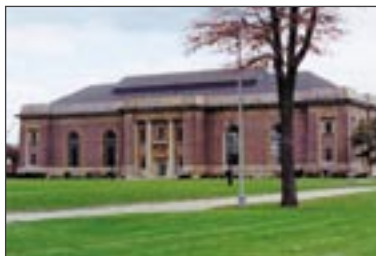
Detroit’s northeastern water plant.
