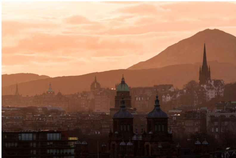
The skyline of the Old and New Towns of Edinburgh World Heritage Site
