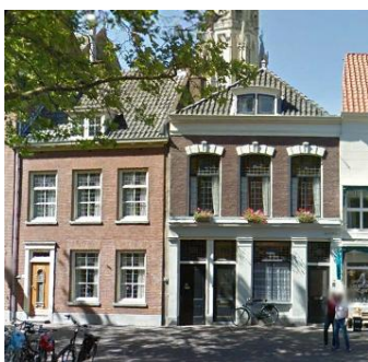
Burgwal no.24-28. The two green doors in the middle are at the spot where the double gate listed in K1667 would have been. BW-E9 is the left house, BW-E10 the right house (excluding the double doors). Obviously the current houses are not 17 th century originals. Source: Google Earth.
