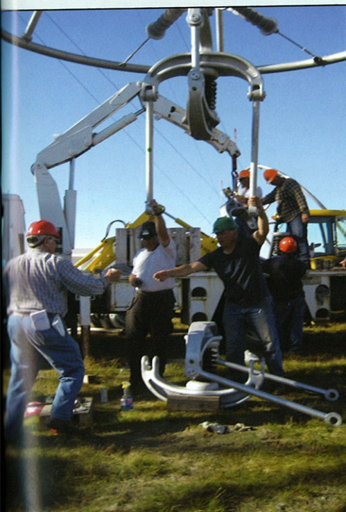
(Background) NCTAMS LANT DET Cutler, ME. (Clockwise from left) Antenna Riggers assemble one of 10 insulator links that make up the fail-safe insulator chain. Riggers install a large corona ring located in the background. A completed fail-safe insulator string.
