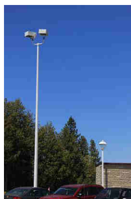
The lighting in Tobermory ferry terminal has been retrofitted to full cut-off lighting.
