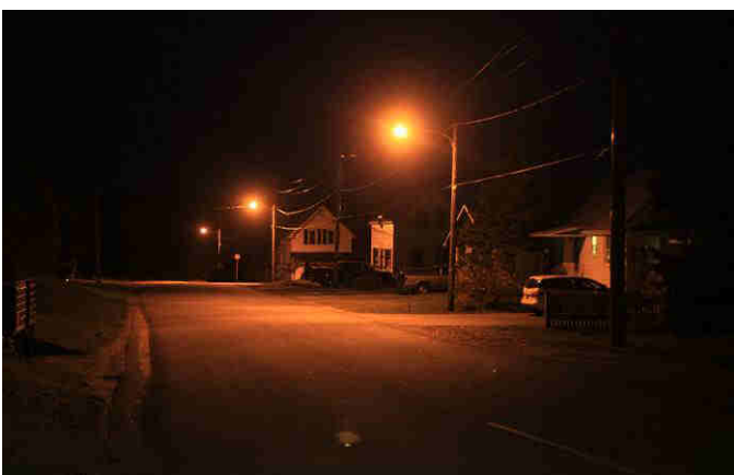
Not full cut-off luminaires with sodium high pressure lamps in side streets Full cut-off LED luminaires in the main street
