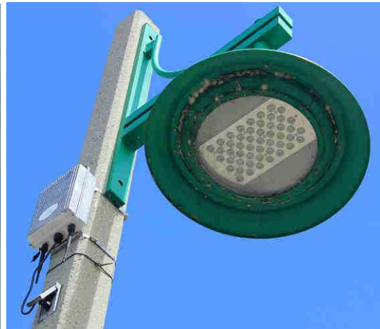
Different types of full cut-off luminaires in use.
